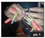
6. The exhaust fan assembly attaches to the top with ten #14 x ½" hex head tap screws. (pic 6a). The wires to the assembly are not numbered and can be fastened either way with the orange wire nuts.
