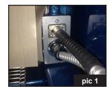
11. The cooler unit's wires are numbered to match up with the wires in the electrical handy box. Remove handy box cover, run the wires and flex conduit into the 90° Romex connector and tighten the screws. Tie the similarly numbered wires together with orange wire nuts (pic 11). Then replace the handy box cover.
